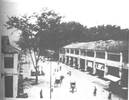
Jalan Kota, Taiping.
